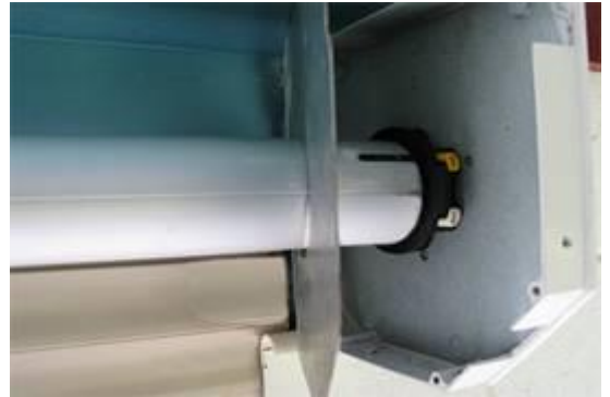
Electric motor on right side of roller shutter.
